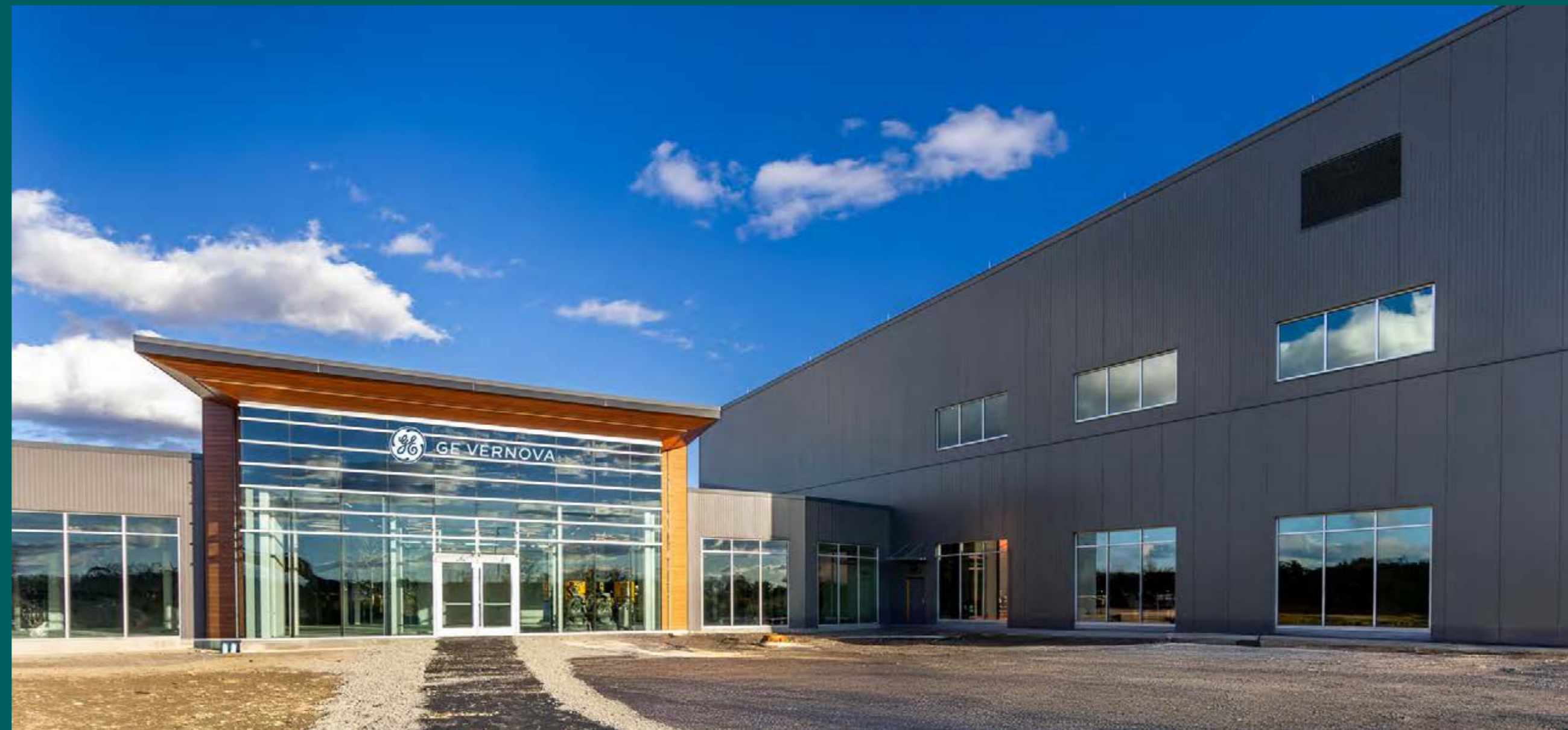
Our new Customer Experience Center and R&D PowerHouse building (home of the 10-ton DAC unit) under construction in Niskayuna, New York.
