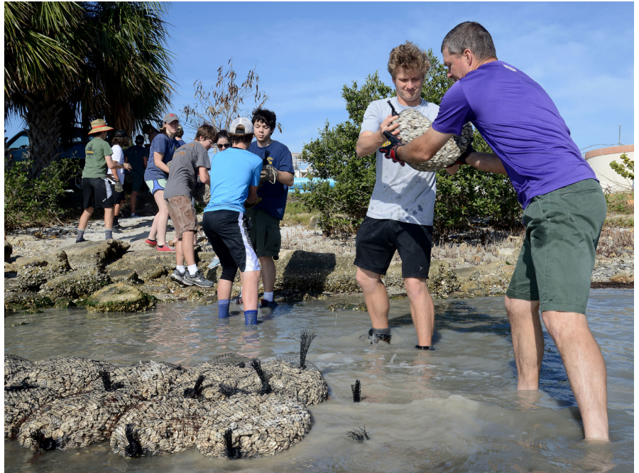
Members of MacDill Air Force Base and the local community build oyster reefs at MacDill Air Force Base, Florida, March 30, 2018. MacDill's eastern shoreline is prone to erosion, however oyster reefs aid in stabilizing the shoreline as well as improving MacDill's vast natural habitats. This build is part of the ongoing Oyster Reef Shoreline Stabilization project, which started in 2004. (Department of the Air Force photo by Staff Sgt Tori Long)
