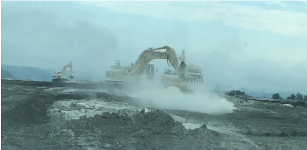
Bucket mixing in use
