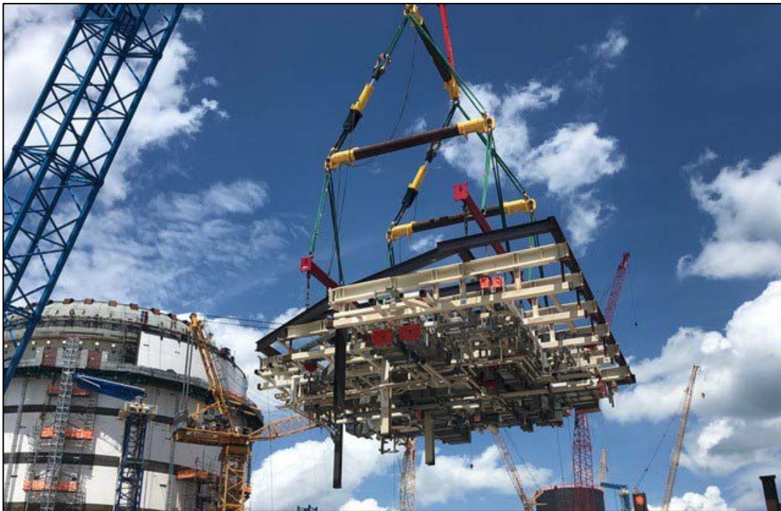
Room 12501 module being set inside the Unit 4 Auxiliary Building
