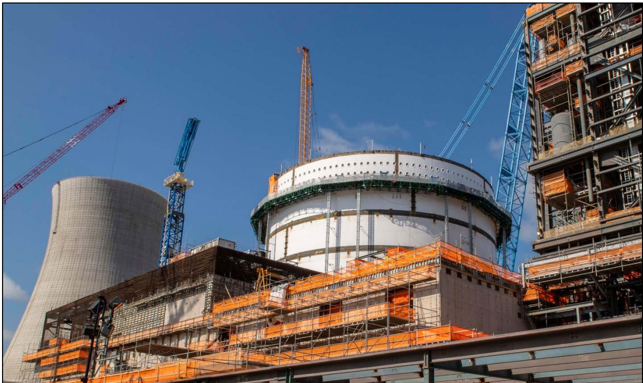
Air Inlet Panels installed on the Unit 4 Shield Building
