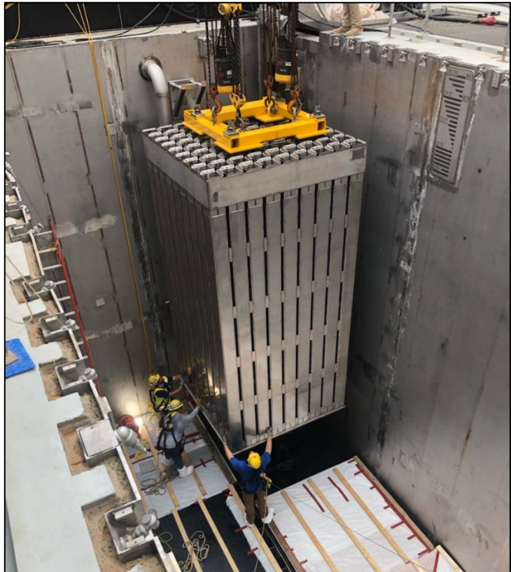
Spent Fuel Rack installation in Unit 3
