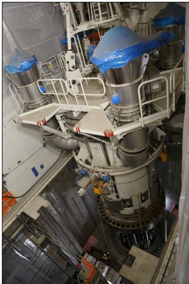
The Integrated Head Package ("IHP") being installed on the Reactor Vessel inside Unit 3 Containment
