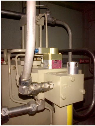
Parker Jet-Pipe ® on Fuel Control Valve
