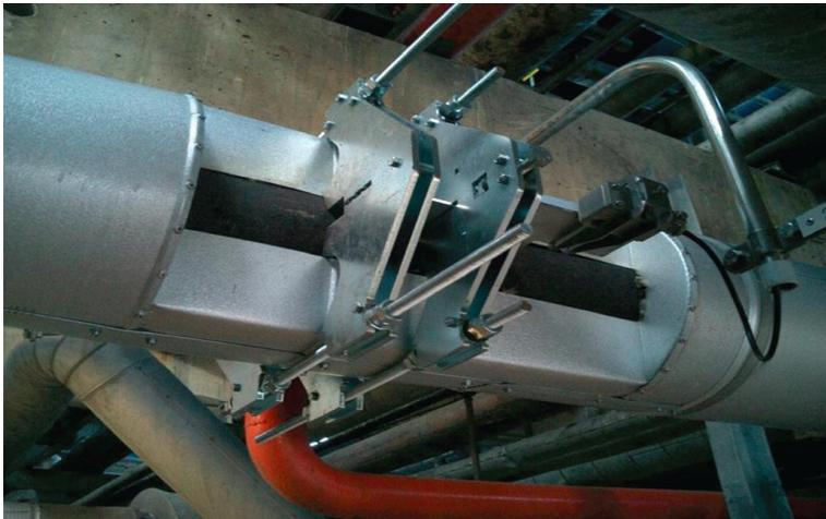
*FLEXIM's clamp-on flow measurement system is designed to stand up to high-temperature applications from -256 F to 750 F.*
